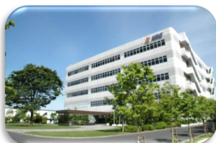
Greened Sayama Plant
